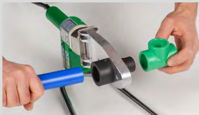
Heating-up of pipe and fitting
