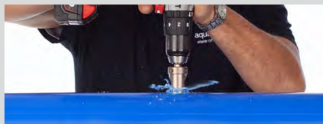
Drilling through the pipe wall
